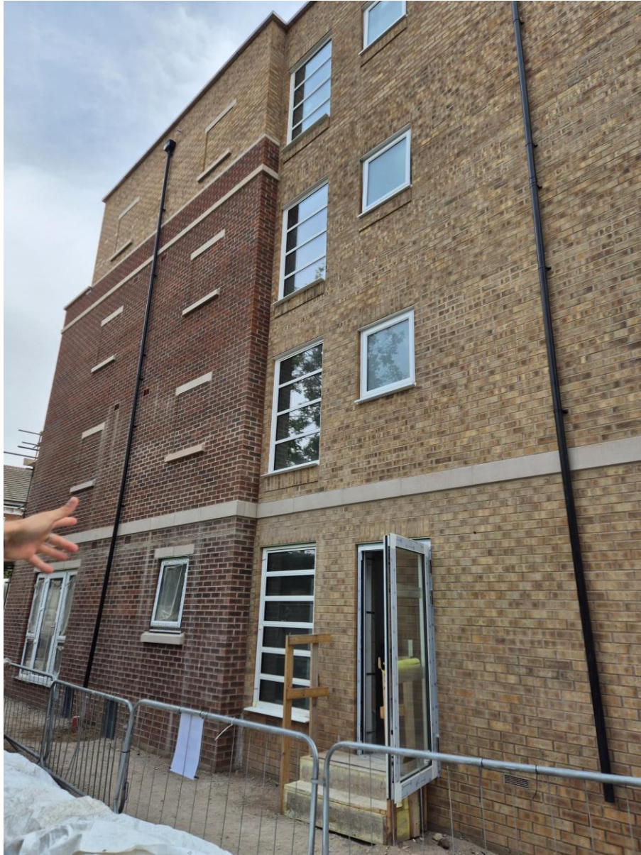
Above: AOV windows to northern elevation
