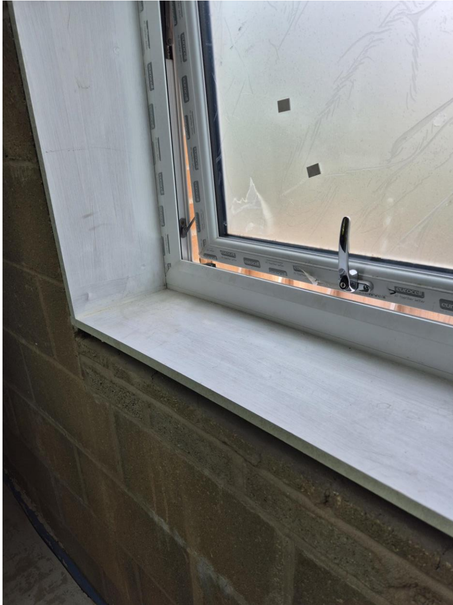
Above: Restrictor to stairwell windows.
